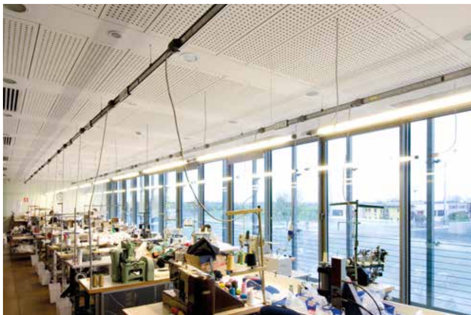
Example of lighting and small power distribution
